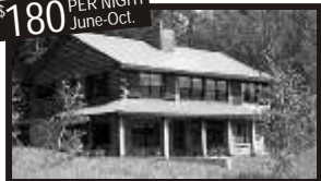
Jack Creek Crew Quarters
